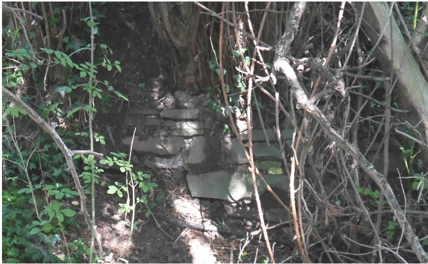
Surviving masonry in the northeast wall.
