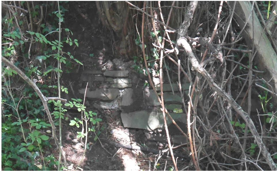
Above, masonry in the northeast wall.
