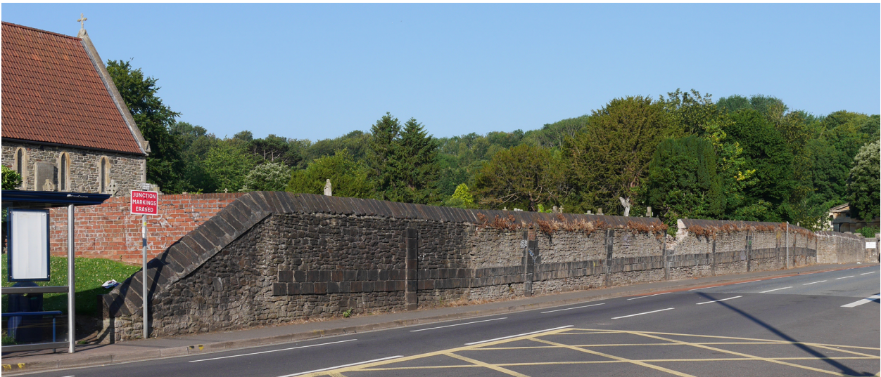
Looking west at the whole of the surviving wall (photo 19 June 2025).
