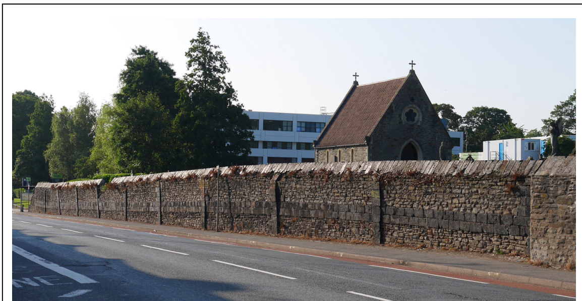
Looking east-southeast at the whole of the surviving wall (photo 19 June 2025).
