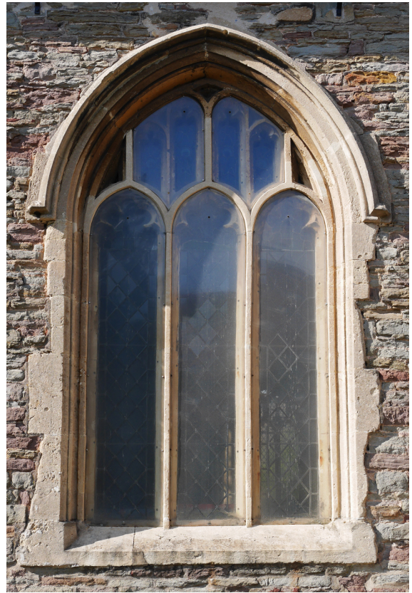
South side of the south aisle, west of the porch (exterior).
