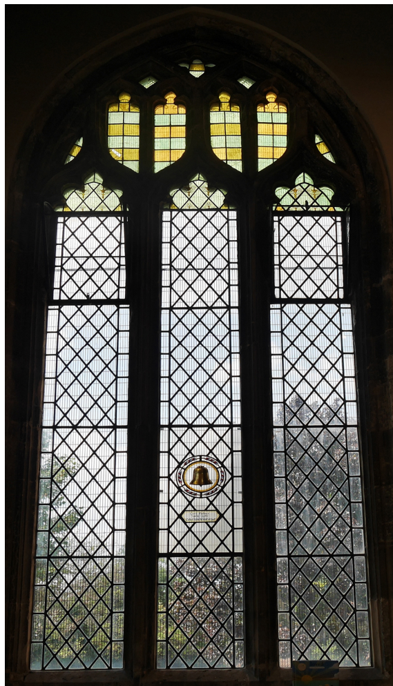
West end of the south aisle (interior).
