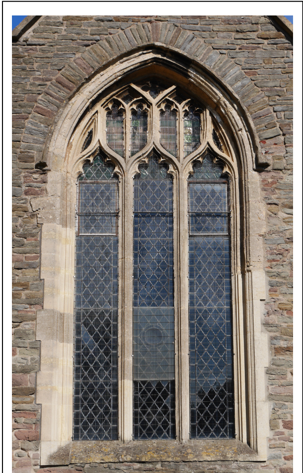
West end of the south aisle (exterior).
