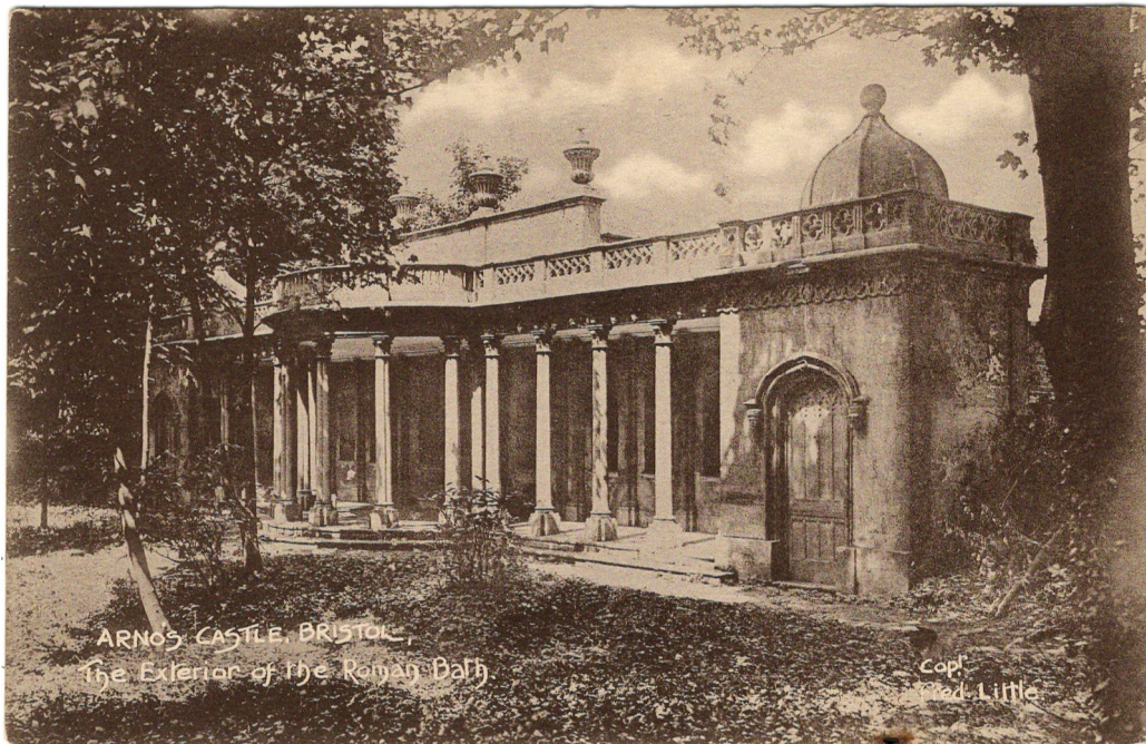
This shows a building lost to Brislington but the façade was moved to the exotic 'village' at Portmeirion, north Wales, where it's known as the Bristol Colonnade. The postcard is titled 'Arno's Castle, Bristol. The Exterior of the Roman Bath.' (it wasn't actually Roman, just in a classical style).
