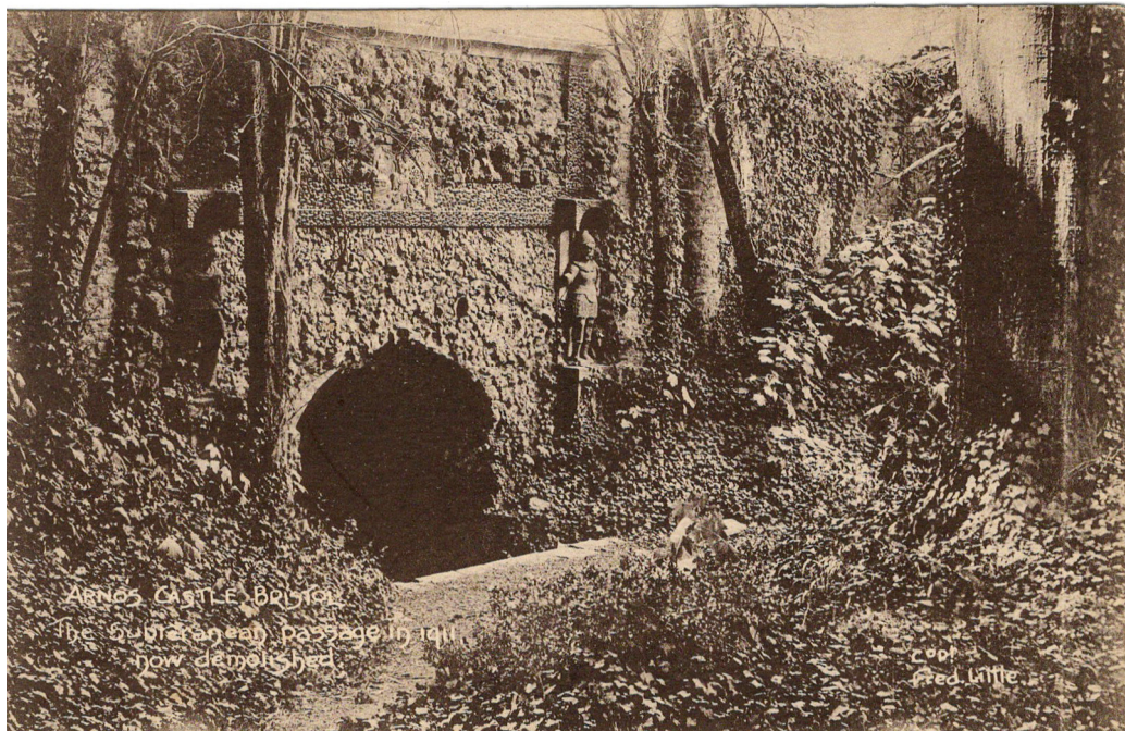
ARNOS CASTLE BRISTOL The Subterranean passage in 1911 now demolished. Copied Fred Little This postcard is titled 'Arno's Castle, Bristol. The Subterranean passage in 1911 now demolished.' This postcard shows an entrance to the tunnel that ran beneath the Bath Road, connecting the house of Arno's Court with the bathhouse and offices/stables at Arno's Castle. Earliest known postmark: 8 November 1912.
