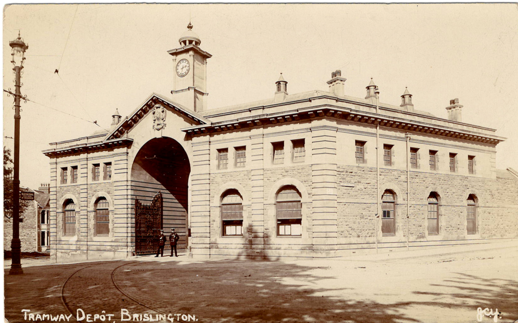
With the title 'TRAMWAY DEPÔT, BRISLINGTON.', this postcard celebrates another key hub in Brislington's transport network. Purpose built as the country's first major depot for electric trams, services began running here in December 1900. This Grade II listed building survives as a prominent landmark on the A4 Bath Road at the junction with Sandy Park Road (on the right of this picture).
