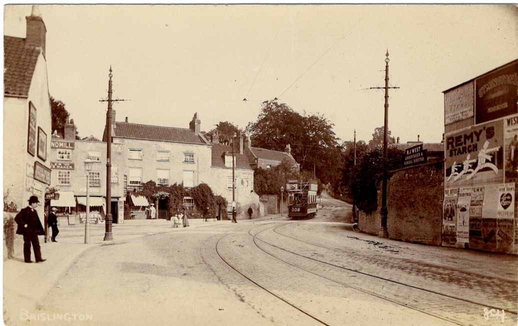
This postcard titled 'BRISLINGTON!' shows a tram at its terminus, pairs of traction poles can be seen, supporting the overhead wires from which the trams drew the electricity for their motors. The largest building in the row beside the tram was Brislington Post Office. On the extreme left-hand side of the postcard, bearing the shadow of the man in the bowler hat, is the wall of the bridge over Brislington Brook.
